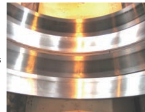
Hardly any indication of rust
