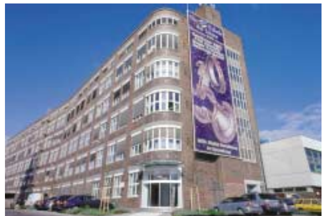
FAG's Aerospace/Super Precision plant in Schweinfurt, Germany
