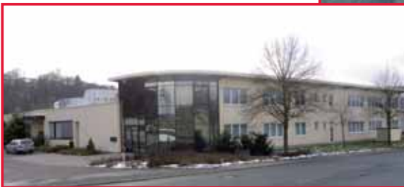
New Plant in Asslar
