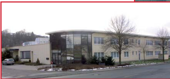
New Plant in Asslar
