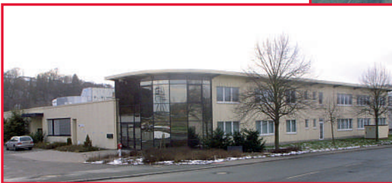
New plant in Asslar
