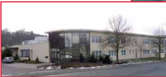
New plant in Asslar
