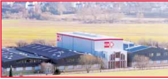
Headquarter of the IBC Wälzlager GmbH at the industrial area of Solms-Oberbiel
