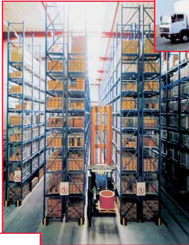
Central Computer Controlled High Shelf Warehouse – Middle 1996
